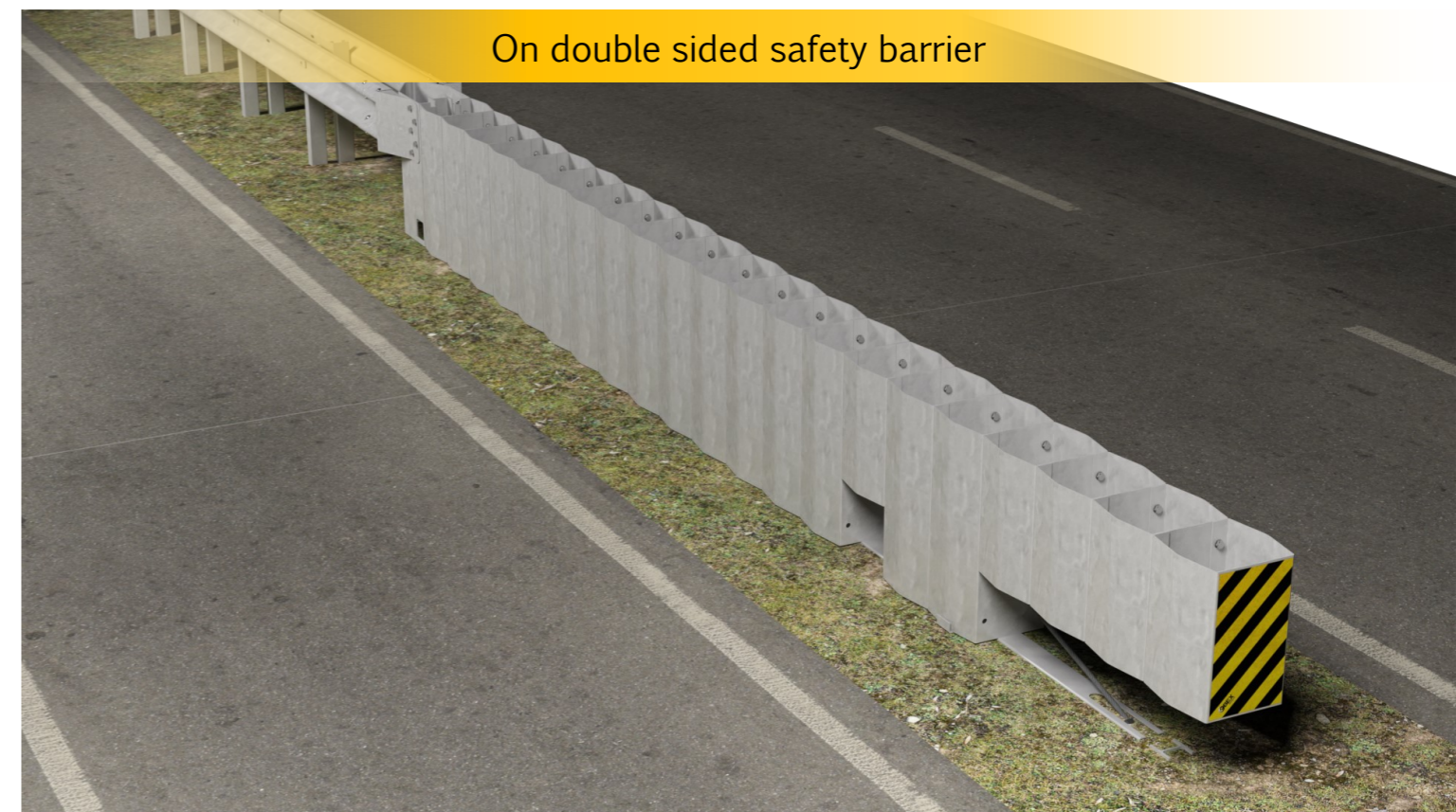
On concrete barrier
